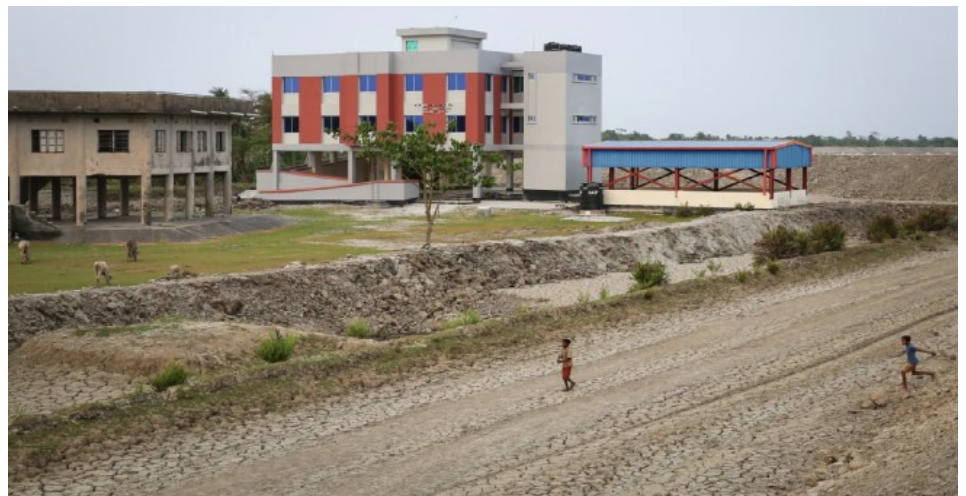
Most cyclone shelters in Bangladesh are also used as schools or community centres. This one in Chila village doubles up as a school (Credit: Catherine Davison)
