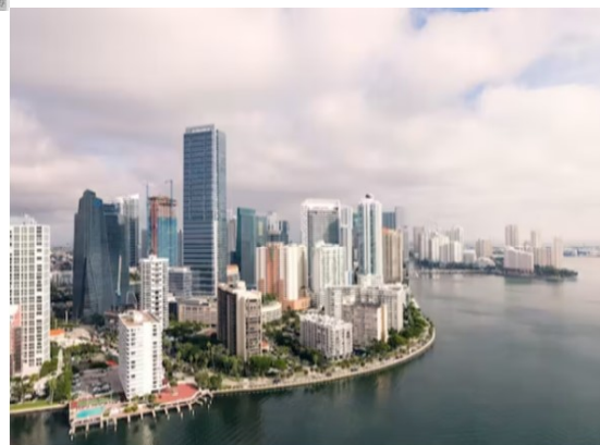
Much of Miami is built right up to the water's edge. On average, it's 6 feet above sea level.
